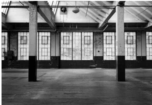
Figure 7. Pre-construction view 1, Nabisco Factory, future site of Dia:Beacon (Riggio Galleries, 1999; photograph, Michael Govan, © Dia Art Foundation).
